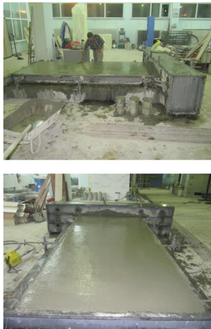
Figure 4. Pouring the concrete of the SW test specimen
