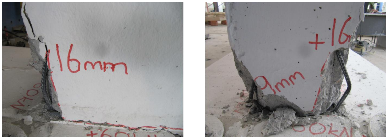
Figure 8. Buckling of longitudinal reinforcements
