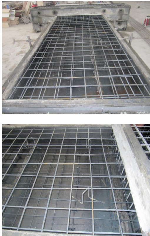
Figure 3. General view of the SW test specimen in the construction stage
